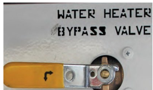
Figure 14-13: Water Heater Bypass System
