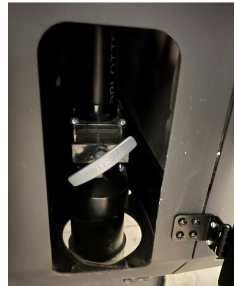
Figure 9-15: Grey Water Gate Valve
