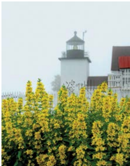
Stockton Springs' Fort Point lighthouse, rebuilt in 1857, points the way to the Penobscot River and Bangor. COURTESY OF VISIT MAINE
