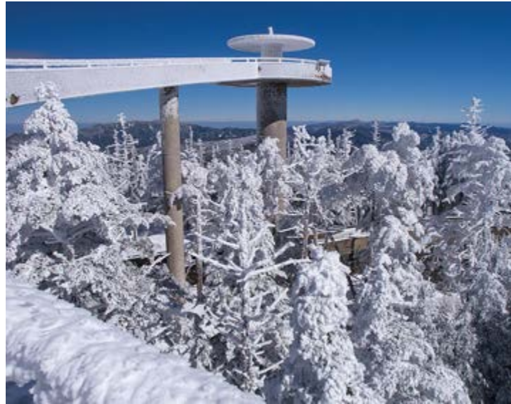
Clingmans Dome Tower dressed in winter white.
