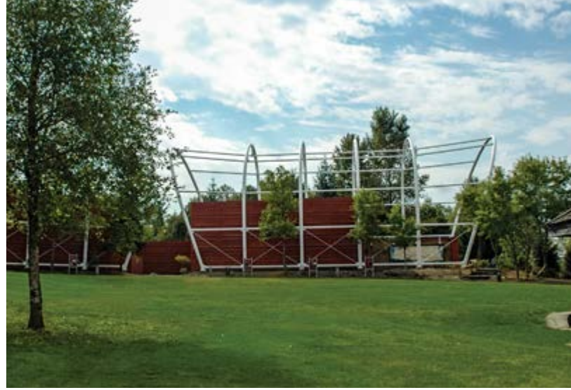
Left: This picture, taken several years ago at the End of the Oregon Trail Interpretive Center, shows the fabric stretched over the frames that simulate the tops of the covered wagons. Above: Now under renovation, the visitor can see the immensity of the frames and the buildings underneath.
