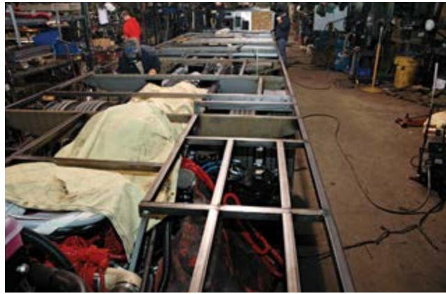
While the Freightliner chassis is in the welding shop, it receives a sturdy steel sub-floor.
