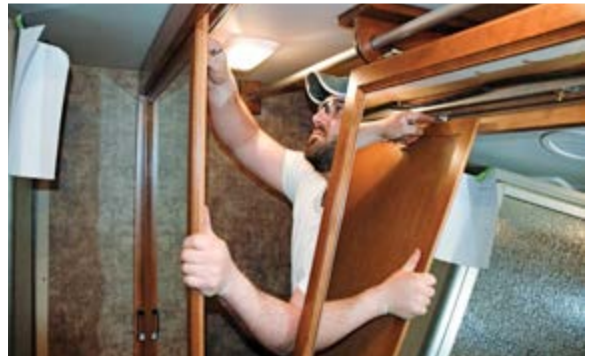
As the motorhome enters its third day on the assembly line, cabinet doors, fascias, and closet doors are installed
