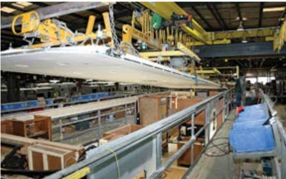
Built in another part of the plant, the roof assembly is lowered into place with an overhead crane.
