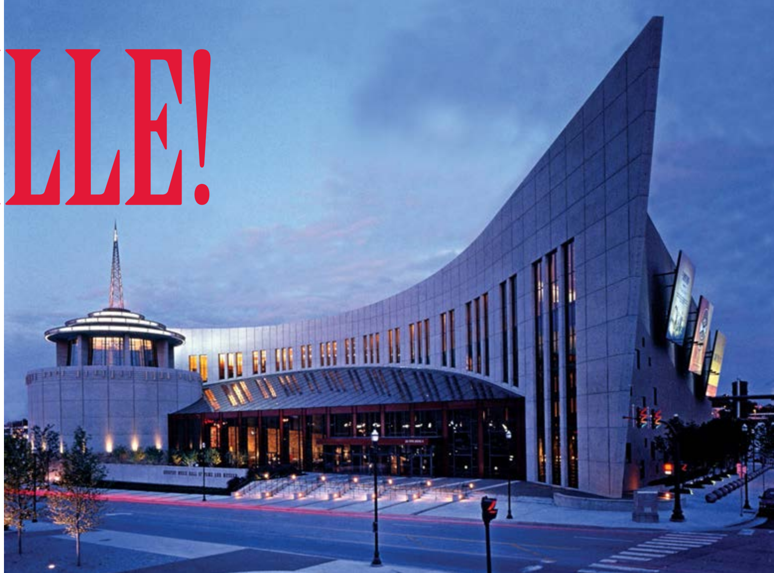
Opened in May 2001, the $37 million structure housing the Country Music Hall of Fame and Museum is very symbolic architecture. The windows resemble black piano keys; the arc on the right side of the
