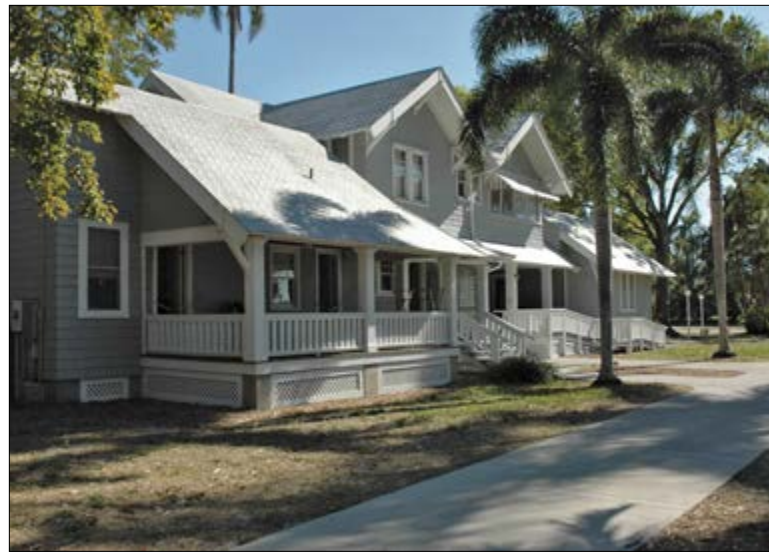
The lumber for Edison's post-and-beam home was cut in Maine and assembled in Ft. Myers. Edison paid $6,700 for the completed house.
