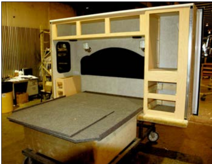
From top to bottom: Cabinet frames and ceiling have been added to this dinette-sofa slide for an Allegro Bay. Ceiling and cabinet frames along with hardware have been added to this Allegro bed slide. A queen-size bed slide for one of the diesel models stands ready to be inserted into the motorhome on the production line. Top right: This bedroom slide houses a lavatory, medicine cabinets, clothes hamper, and ample storage for clothing.
