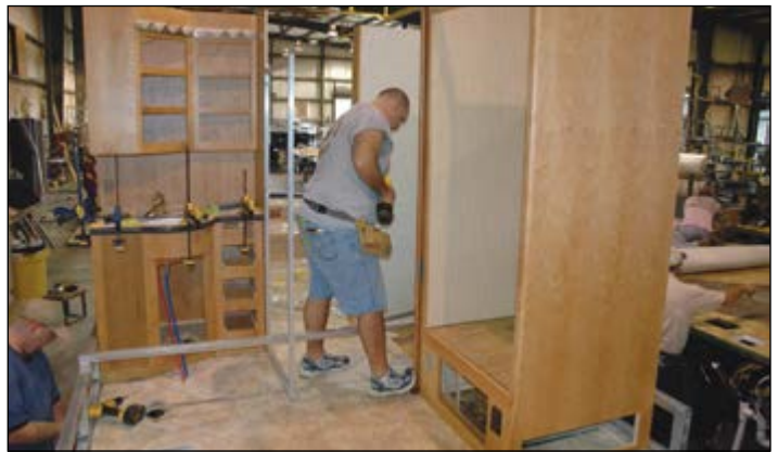
At Station 4 cabinets and partitions are perfectly aligned with jigs and frames to hold them in position until the sidewalls are installed.
