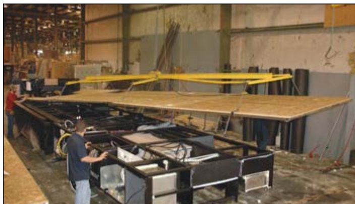
Built as a sub-assembly, the entire floor is installed at Station 2.
