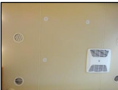
Figure 0-3: Typical Ceiling in the BYWAY
