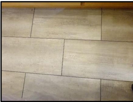
Figure 0-2: Typical Flooring in the BYWAY
