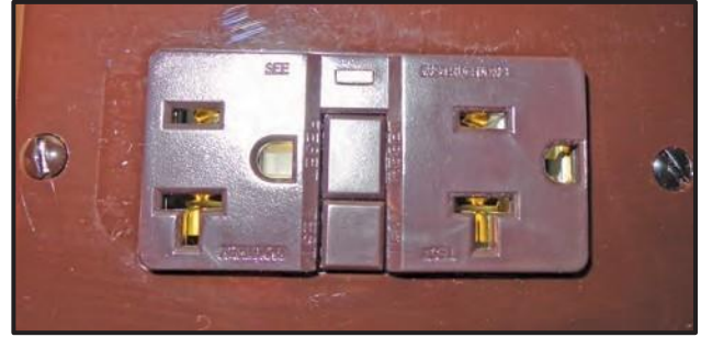
Figure 0-6: GFCI Receptacle
