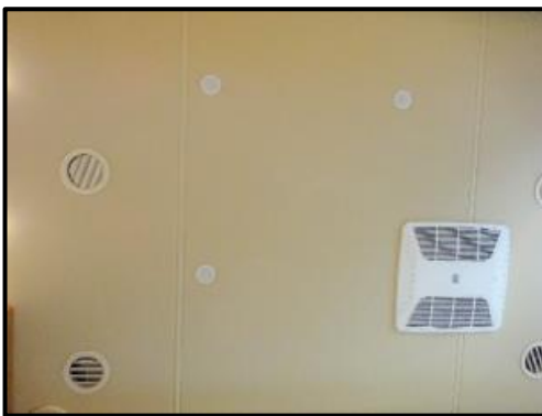
Figure 0-3: Typical Ceiling in the BYWAY
