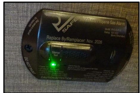
Figure 0-5: Carbon Monoxide/LP Gas Detector
