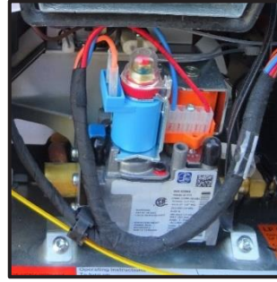
Figure 0-9: Water Heater Relief Valve
