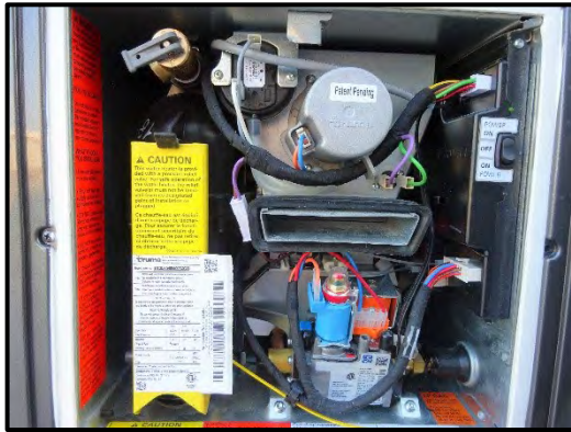
Figure 5-7: Water Heater
