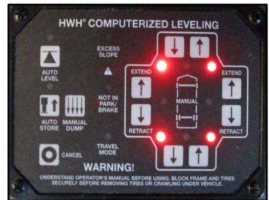
Figure 15-6: HWH Control Panel
