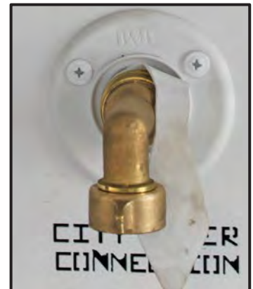
Figure 13-8: City Water Supply Connection
