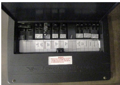
Figure 9-5: 120 VAC Circuit Breaker Box
