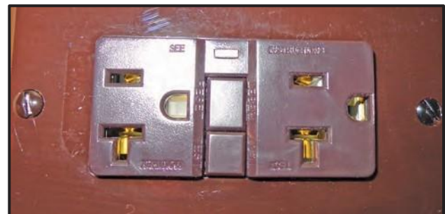
Figure 8-15: GFCI Receptacle
