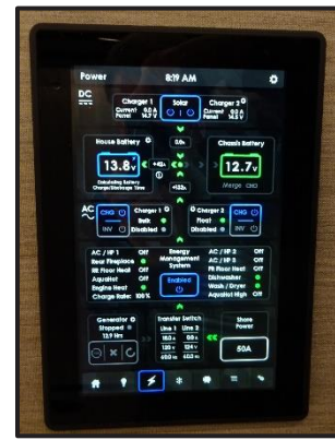
Figure 8-17: Energy Management System
