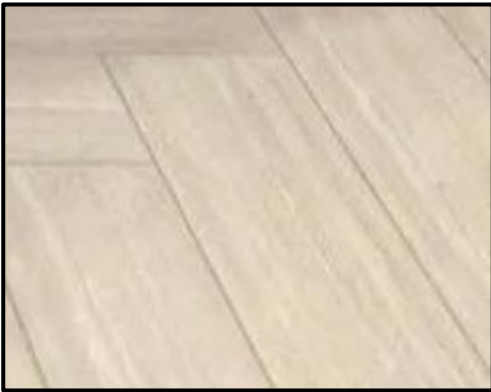
Figure 11-2: Typical Flooring in the Zephyr
