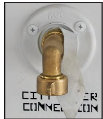
Figure 12-7: City Water Supply Connection
