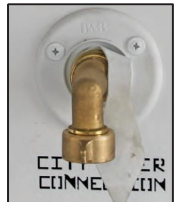
Figure 12-7: City Water Supply Connection
