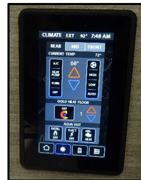
Figure 11-3: Heated Tile Floor Controller
