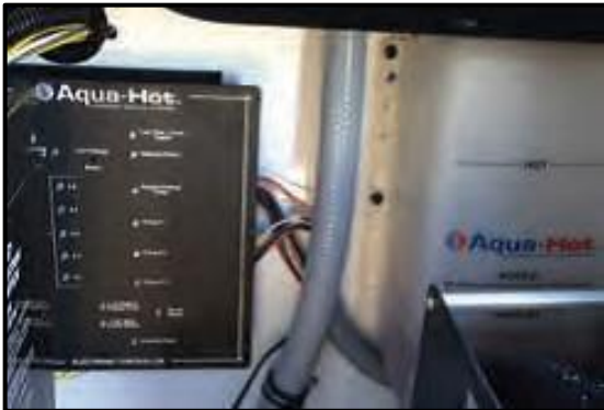
Figure 12-15: Aqua-Hot Heating System
