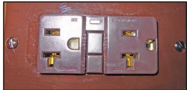
Figure 8-14: GFCI Receptacle
