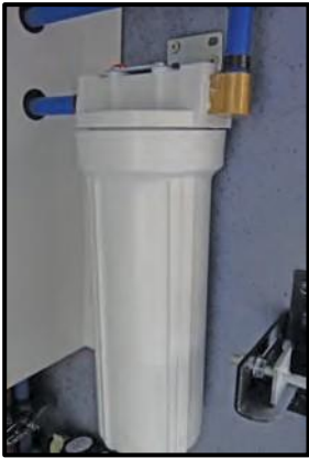
Figure 12-8: Water Filter
