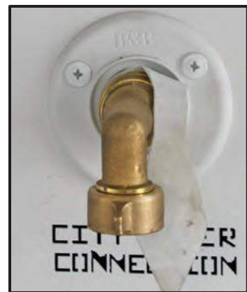
Figure 12-6: City Water Supply Connection
