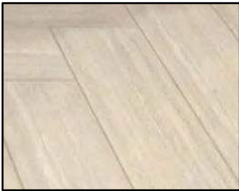
Figure 11-2: Typical Flooring in the Zephyr
