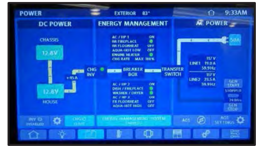
Figure 8-15: Energy Management System
