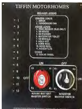
Figure 8-5: House Battery Disconnect Panel Switch
