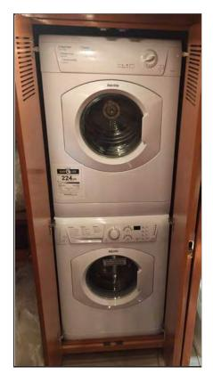
Figure 4-7: Stacked washer/dryer
