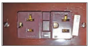
Figure 8-13: 120 VAC GFCI receptacle
