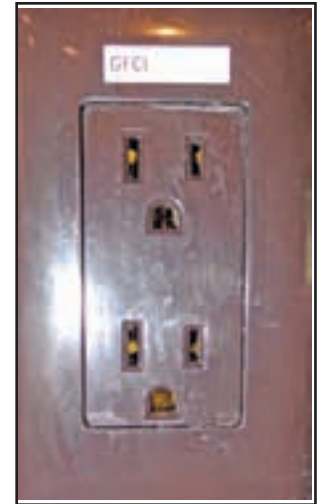
Figure 8-12: 120 VAC receptacle
