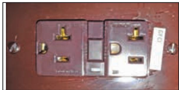
Figure 8-13: GFCI receptacle
