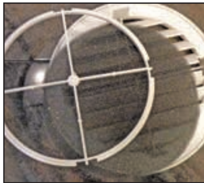
Figure 3-5: Round vent filter
