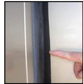
Figure 14-6. Inspecting Slide Out Gasket
