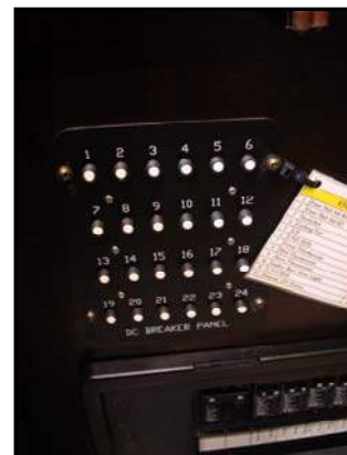
Figure 7-18 Resettable Circuit Breakers
