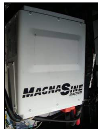
Figure 7-14. Sine Wave Inverter
