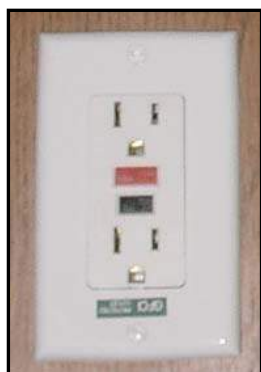
Figure 7-13. Ground-Fault Circuit Interrupter (GFCI)
