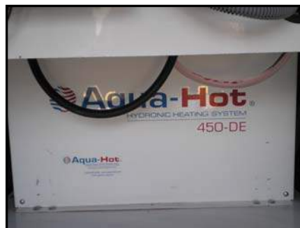
Figure 3-2. Hydraunic Heating System
