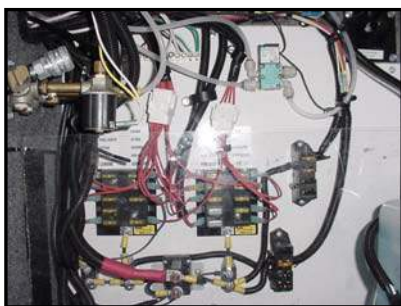
Figure 7-4. 12 VDC Fuse Panels
