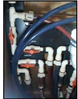
Figure 11-9. Plumbing Manifold
