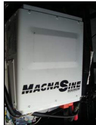
Figure 7-14. Sine Wave Inverter
