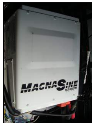
Figure 7-14. Sine Wave Inverter
