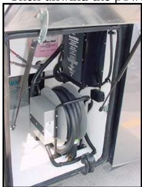
Figure 7-2. Electrical Power Hookup Cable
