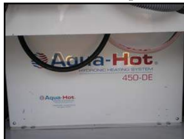
Figure 4-10. Hydraunic Heating System
