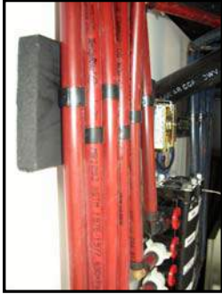
Figure 11-9. Plumbing Manifold
