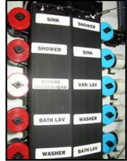
Figure 11-10. Plumbing Manifold
