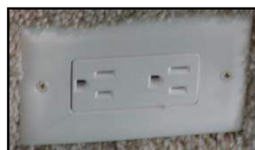
Figure 7-11. 120 VAC Outlets
