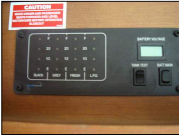
Figure 11-1. Monitor Panel (Water, LP Gas, Battery)
