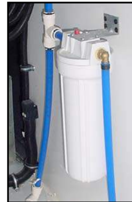
Figure 11-9. Water Filter
