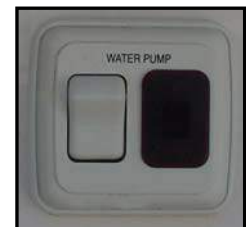
Figure 11-6. Water Pump Switch
