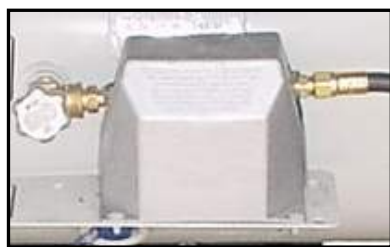
Figure 2-6. LP Gas Regulator
