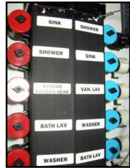
Figure 11-11. Plumbing Manifold
