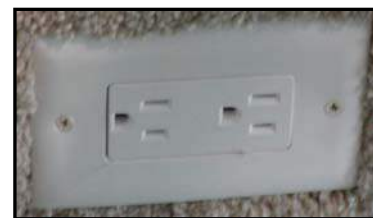
Figure 7-10. 120 VAC Outlets
