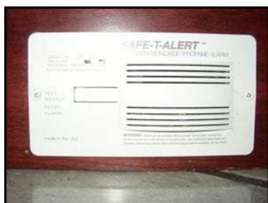
Figure 4-20. Carbon Monoxide/ LP Gas Combination Detector
