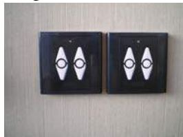
Figure 10-6. Control for Passenger & Entry Door Power Shades
