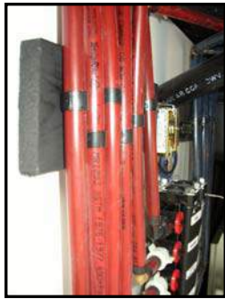
Figure 11-10. Plumbing Manifold
