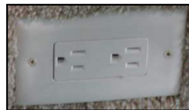
Figure 7-10. 120 VAC Outlets
