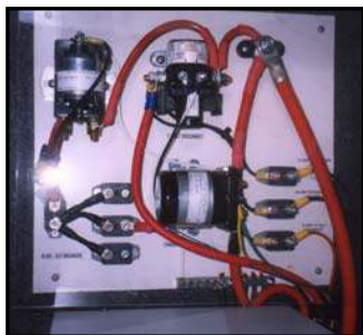
Figure 7-18. Resettable Circuit Breakers
