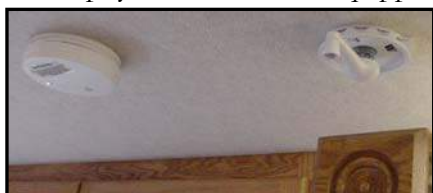
Figure 2-7. Smoke Detector (Left)
