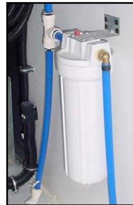
Figure 11-9. Water Filter
