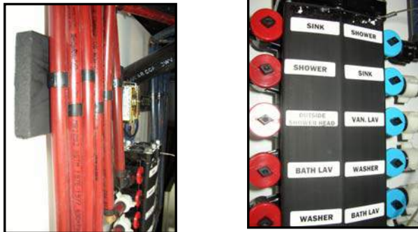
Figure 11-11, 12. Plumbing Manifold
