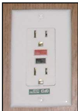
Figure 7-12. Ground-Fault Circuit Interrupter (GFCI)
