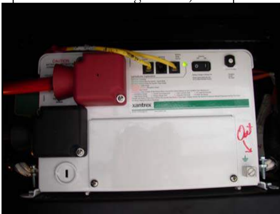
Figure 7-14. Inverter/Converter
