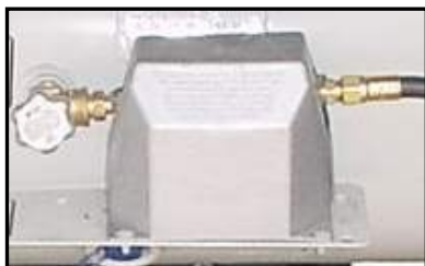
Figure 2-5. LP Gas Regulator
