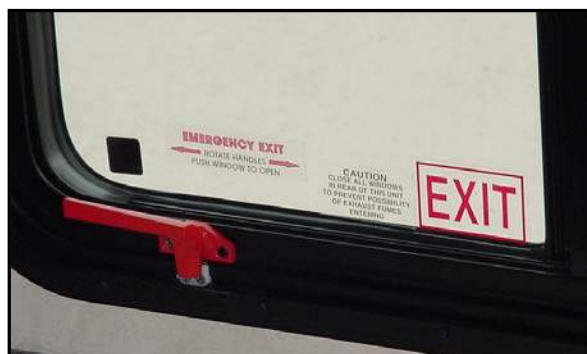
Figure 2-8. Emergency Exit Window
