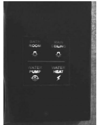
Figure 5-3: Water Heater Controls
