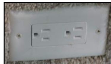
Figure 7-10. 120 VAC Outlets
