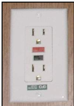
Figure 7-12. Ground-Fault Circuit Interrupter (GFCI)
