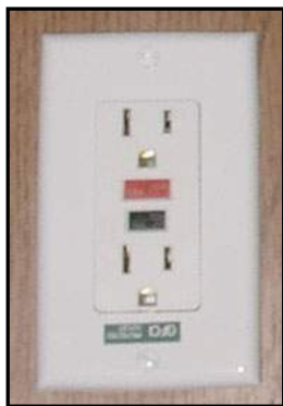
Figure 7-11. Ground-Fault Circuit Interrupter (GFCI)
