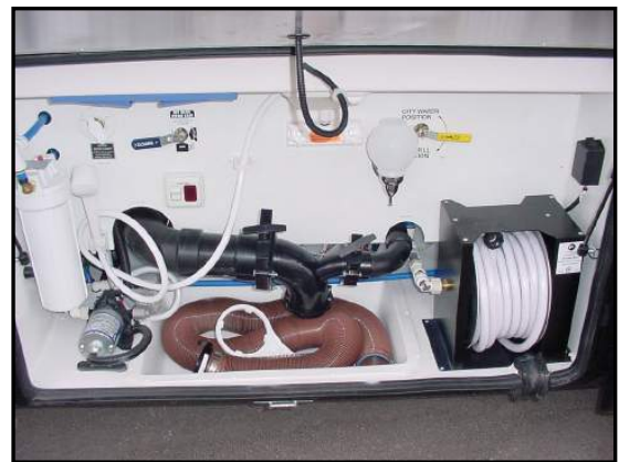
Figure 11-17. Exterior Shower in Outside Compartment
