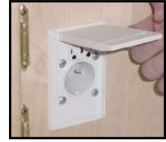
Figure 14-5. Vacuum Hose Coupling
