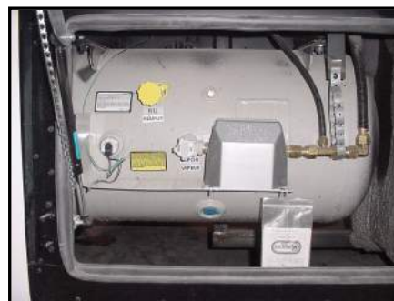
Figure 2-4. Liquid Propane Tank
