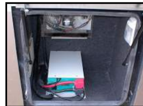
Figure 7-13. Inverter/Converter
