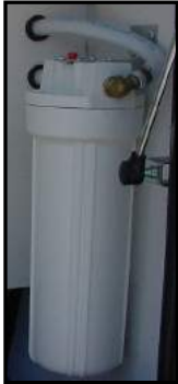
Figure 11-8. Water Filter
