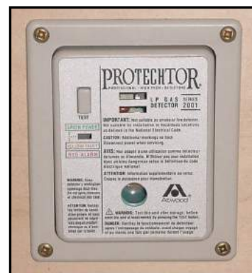
Figure 3-4. LP Gas Detector
