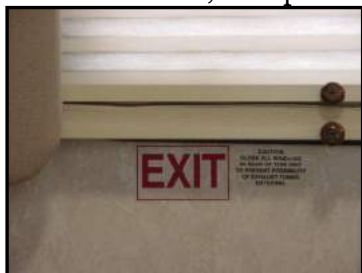
Figure 13-1. Emergency Exit Window
