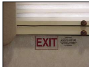
Figure 2-7. Emergency Exit Window
