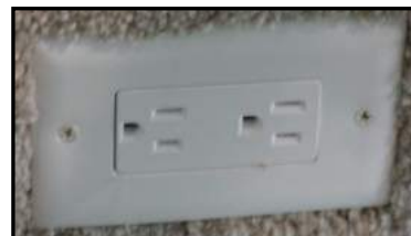
Figure 7-9. 120 VAC Outlets
