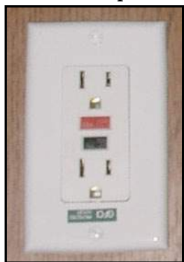
Figure 7-11. Ground-Fault Circuit Interrupt (GFI)
