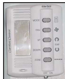
Figure 3-2. Thermostat
