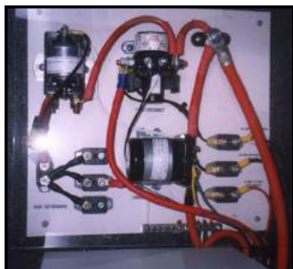
Figure 7-18. Resettable Circuit Breakers
