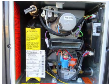
Figure 5-3: LP Water Heater
