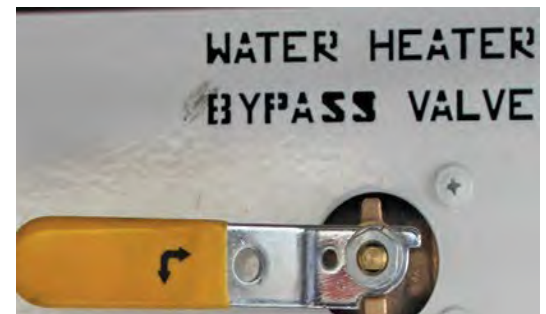
Figure 14-13: Water Heater Bypass System
