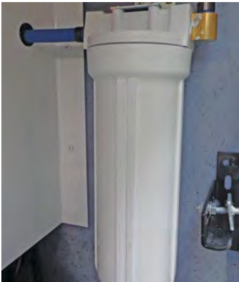
Figure 14-12: Water Filter
