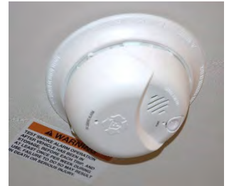
Figure 2-6: Smoke Detector
