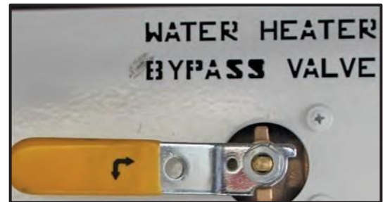
Figure 15-10: Water Heater Bypass System
