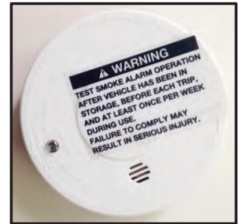
Figure 18-11: Smoke Detector
