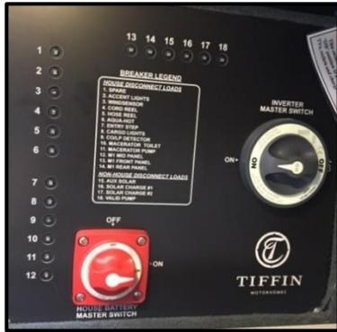
Figure 11-4: House Battery Disconnect Panel
