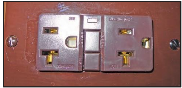
Figure 11-11: GFCI Receptacle
