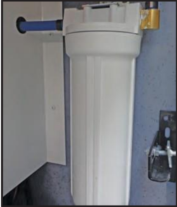
Figure 15-9: Water Filter
