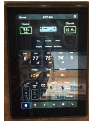
SPYDER Control showing approximate amount of LP Gas Remaining in Tank.
