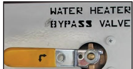
Figure 14-10: Water Heater Bypass System
