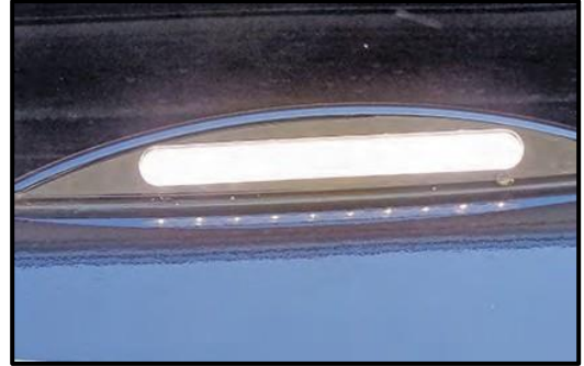
Figure 12-3: Exterior Security Light
