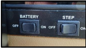
Figure 10-6: 12 VDC Disconnect Switch
