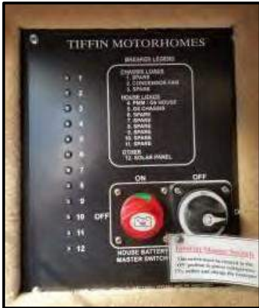
Figure 10-5: House Battery Disconnect Panel
