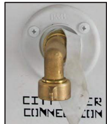
Figure 14-8: City Water Supply Connection
