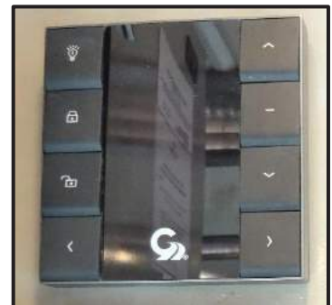
Figure 15-3: Patio Awning Control Switch
