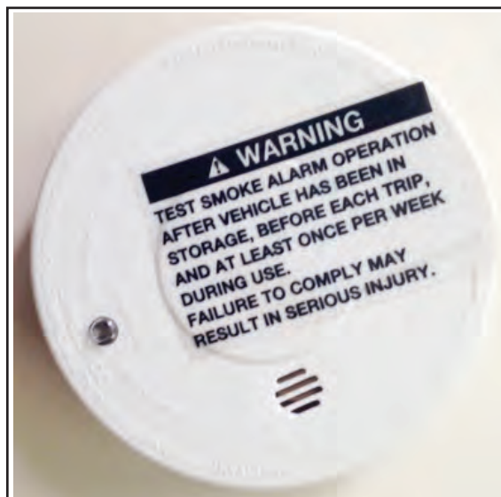
Figure 2-7: Smoke detector.
