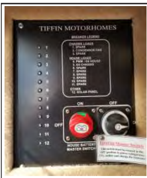
Figure 10-5: House battery disconnect panel switch
