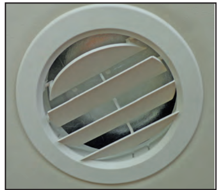
Figure 4-6: Round air vent
