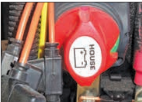
Figure 9-5: House battery disconnect panel switch
