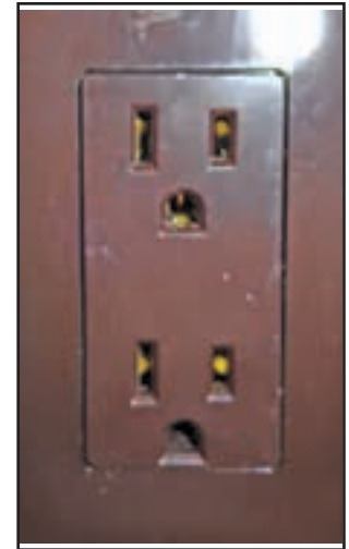
Figure 9-12: 120 VAC receptacle
