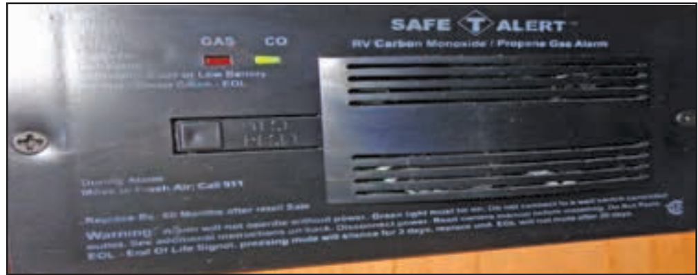
Figure 2-5: Carbon Monoxide alarm
