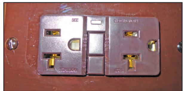
Figure 9-13: GFCI receptacle
