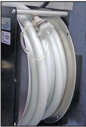
Figure 13-6: City water supply connection
