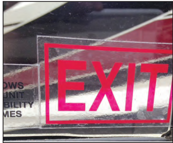
Figure 2-9: Emergency exit window
