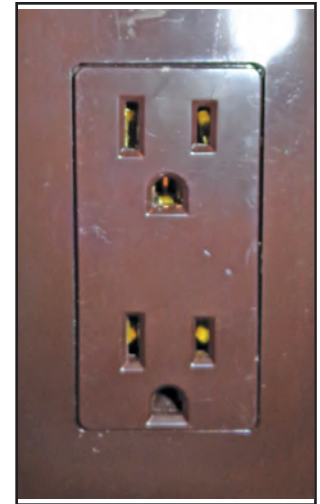
Figure 9-12: 120 VAC receptacle
