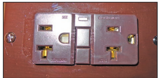
Figure 9-13: GFCI receptacle
