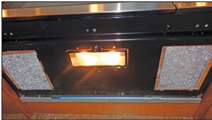
Figure 5-4: Air filtration fans
