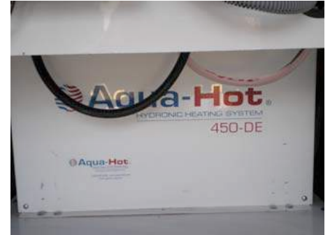
Figure 4-18. Hydraulic Heating System
