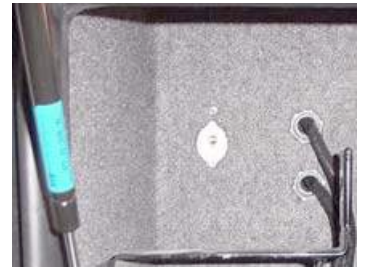
Figure 4-8. Cable & Telephone Jack
