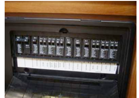
Figure 7-14. Circuit Breakers
