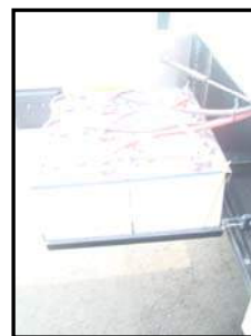
Figure 7-6. Batteries on Slide Tray
