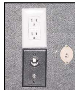
Figure 7-9. 12 VDC Receptacle (black)
