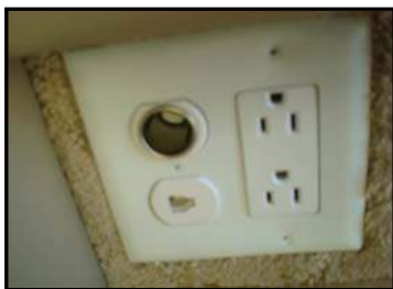
Figure 7-8. 120 VAC Receptacle
