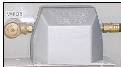
Figure 2-6. LP Gas Regulator
