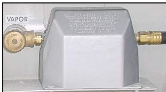
Figure 3-5. LP Gas Regulator
