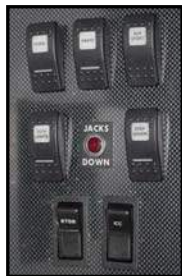
Figure 7-3. Auxiliary Start Switch
