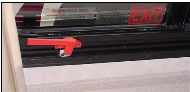
Figure 13-2. Bedroom Emergency Exit Window
