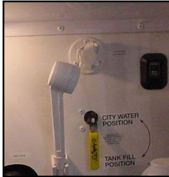
Figure 11-7. City Water Supply Connection
