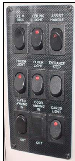
Figure 7-8. 12 VDC Disconnect Switch
