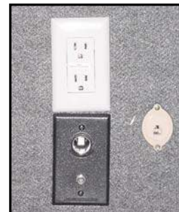
Figure 7-10. 12 VDC Receptacle (black)
