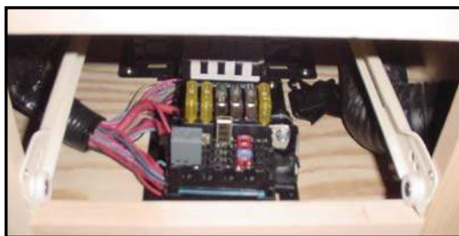
Figure 7-21. Fuse Blocks within Center Console
