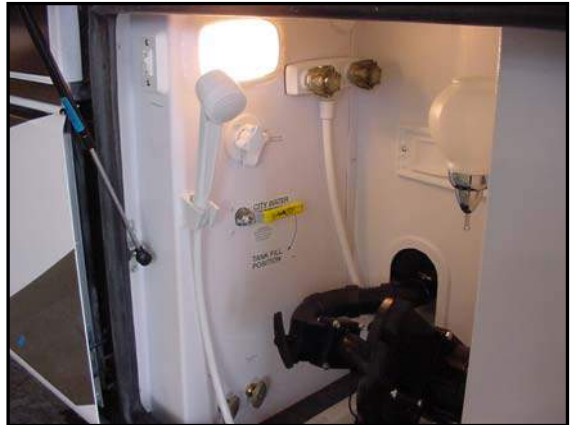
Figure 11-12. Exterior Shower and Exterior Light
