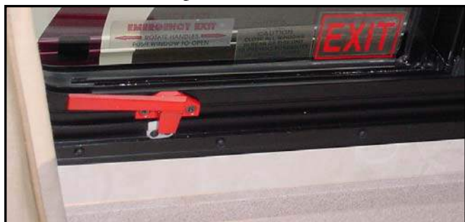
Figure 13-2. Bedroom Emergency Exit Window
