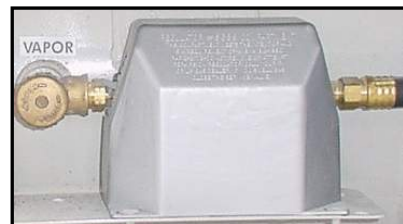
Figure 2-5. LP Gas Regulator
