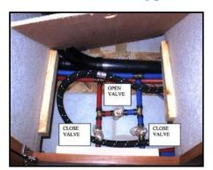
Figure 11-8. Water Heater Bypass System
