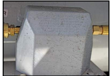
Figure 4-2: LP Gas Regulator
