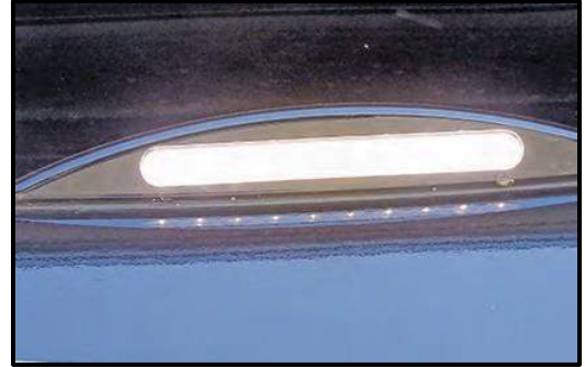
Figure 11-3: Exterior Security Light
