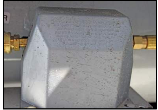
Figure 2-4: LP Gas Regulator
