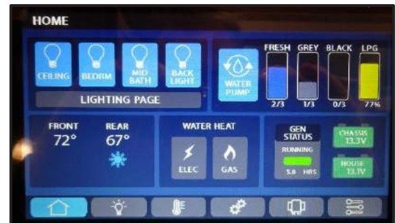
Figure 13-5: Spider Controls System Switch
